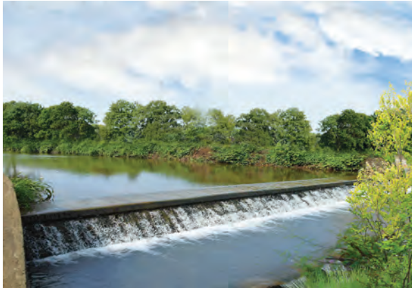
2.3.9 Concrete cement stream check dams
